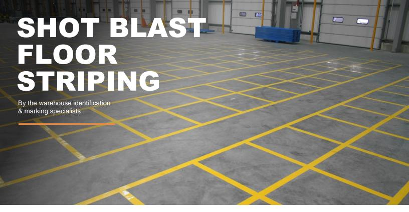
Preparing the concrete prior to applying a paint system is fundamentally important to the performance and longevity of warehouse floor striping. The term 'Shot Blast' is used to describe the method of preparation used on concrete, before applying paint.
