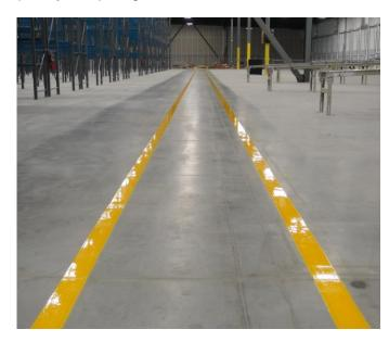
Our specialist machines are used to remove the top surface of a concrete floor, using diamond cutting technology which 'shaves' away  $\frac{1}{8}$ " deep and 4" wide of concrete, creating a channel. The purpose of this is to expose fresh concrete for the paint to adhere to, as well as allowing the paint to sit flush or just below the floor surface level.
