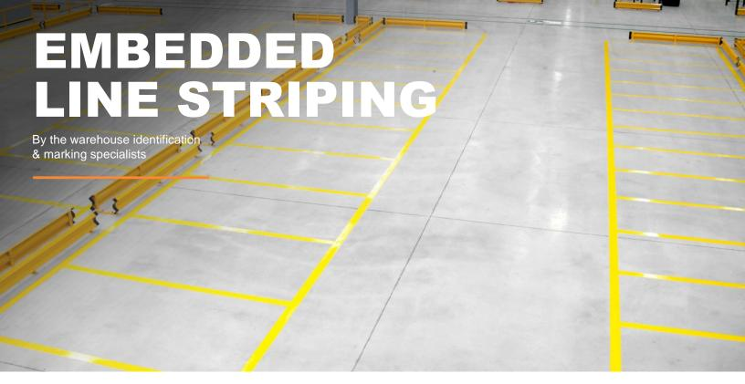
Embedded floor striping is the choice of building owners and long terms tenants of distribution centers. Embedded is the most durable and permanent available. Advanced diamond blade technology used to prepare the concrete prior to applying paint, is extremely accurate and makes the lines exceptionally tough.
