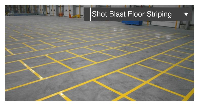
Preparing the concrete prior to applying a paint system is fundamentally important to the performance and longevity of warehouse floor striping. The term 'Shot Blast' is used to describe the method of preparation used.
